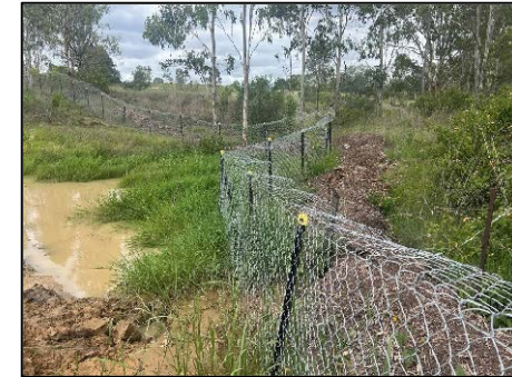
Photo set 5: Temporary Fauna Exclusion Fencing 2023
