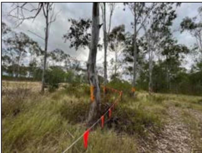
Photo Set 1: Temporary fauna friendly tree protection fencing.
