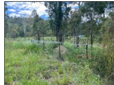
Photo set 6: Temporary Fauna Exclusion Fencing 2024
